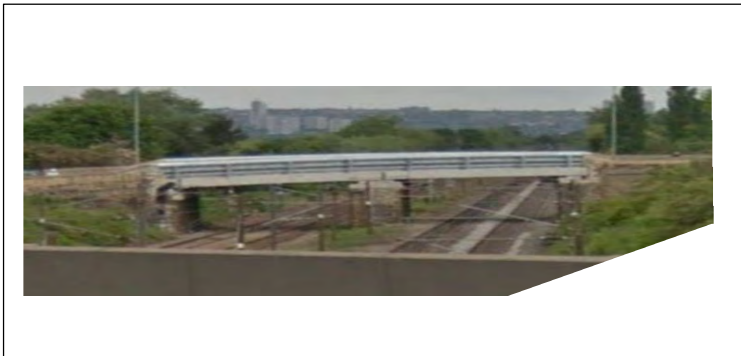
Figure 1 - Photograph of Chowdene Bank Bridge – located north of the existing Allerdene Bridge
